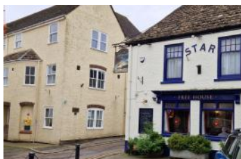
Crown House opposite Star Market Street W3W //skewed.mallets.pill
